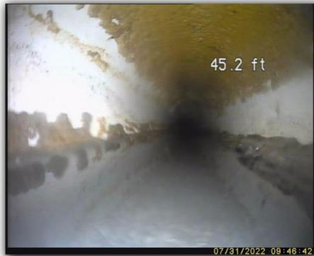
✗ There is an obstruction/blockage in the drain pipe at one or more locations
