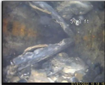
✗ Toilet paper was observed in the drain line at one or more locations. This can be indicative of negative slope or rust/scaling buildup within the pipe. As a result, clogs may develop from time to time.
