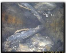
X Toilet paper was observed in the drain line at one or more locations. This can be indicative of negative slope or rust/scaling buildup within the pipe. As a result, clogs may develop from time to time.
